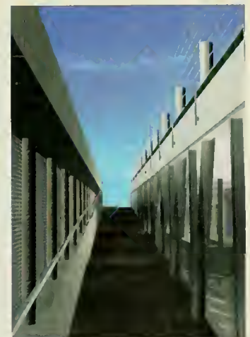
View looking back through entry ramp.
